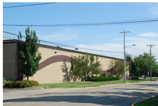
Neenah Water Filtration Plant
