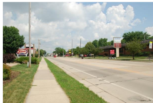
South Commercial Street Business Corridor
