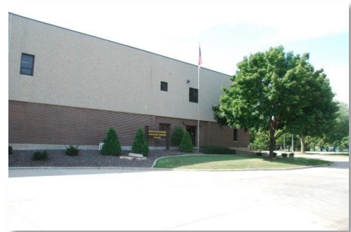
Neenah-Menasha Sewerage Commission WWTf
