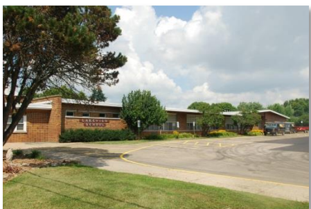
Lakeview Elementary School
