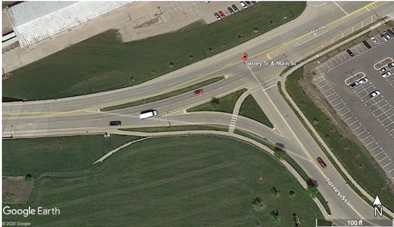
Figure 1: Existing Main Street Intersection with Torrey Street
