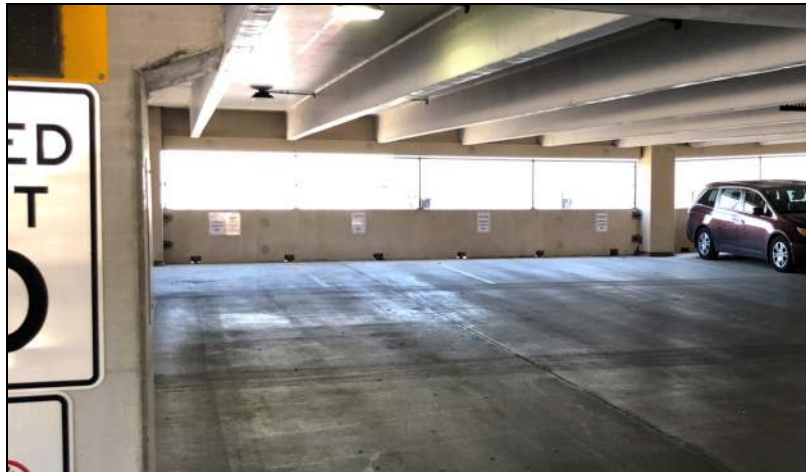
Figure 5: Northwest corner of existing parking ramp
