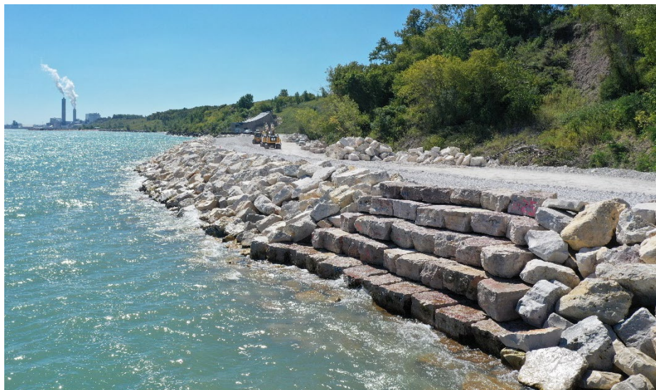
Figure 6. Terrace stone water touch point included along a revetment.
