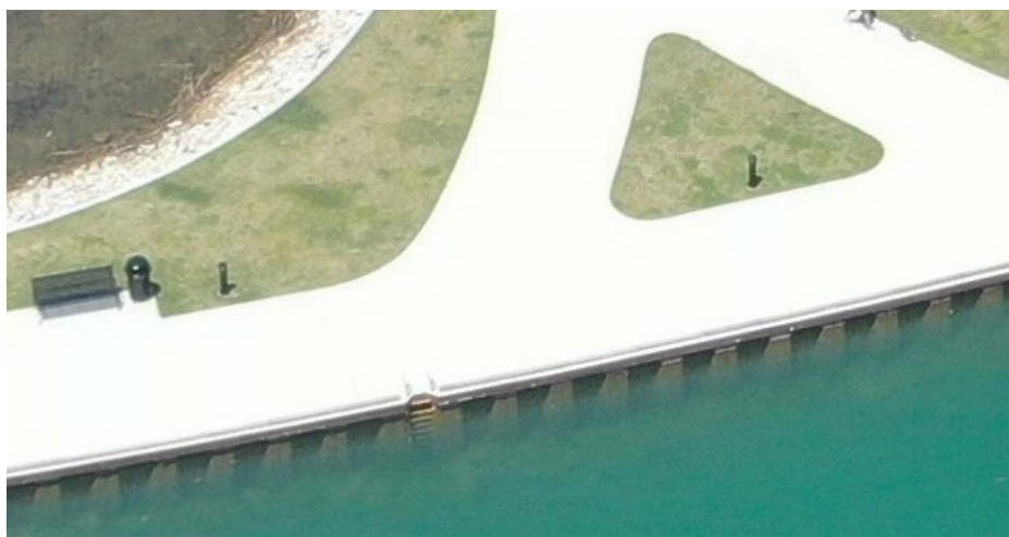
Figure 5. Sheet pile face with concrete decking.
