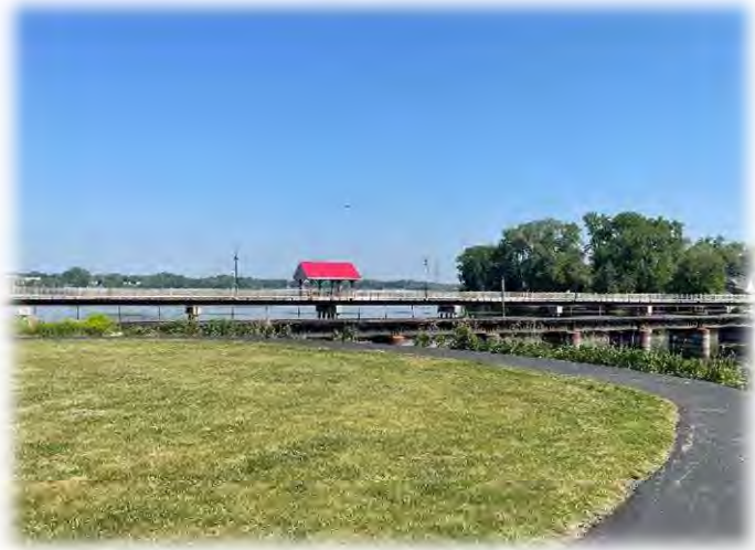
Loop the Lakes Trail from Arrowhead Park Trestle - Plexus
