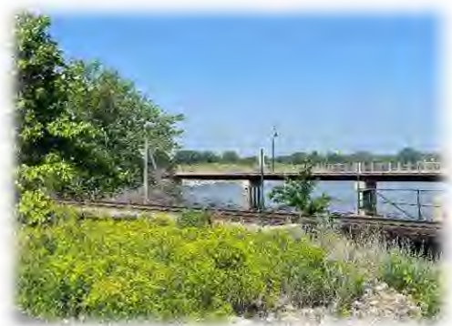
Arrowhead trestle connection
