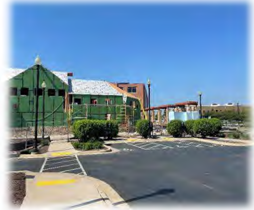
Gateway Plaza Ice Skating Rink construction
