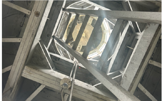
Existing lighthouse catwalk prior to construction.
