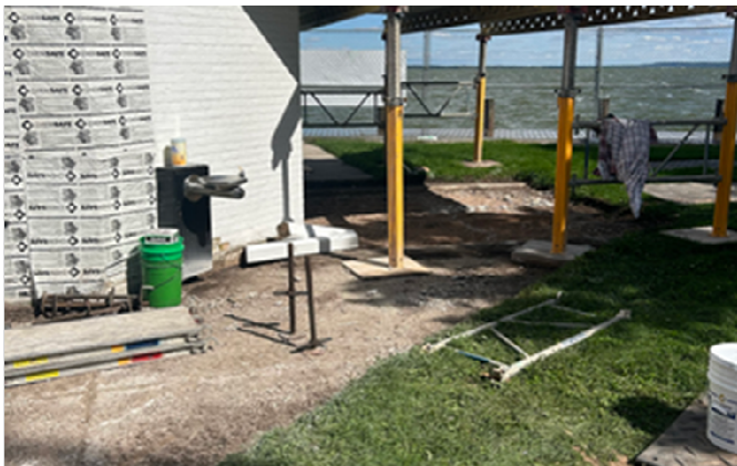
Shoring of bathroom canopies for replacement.
