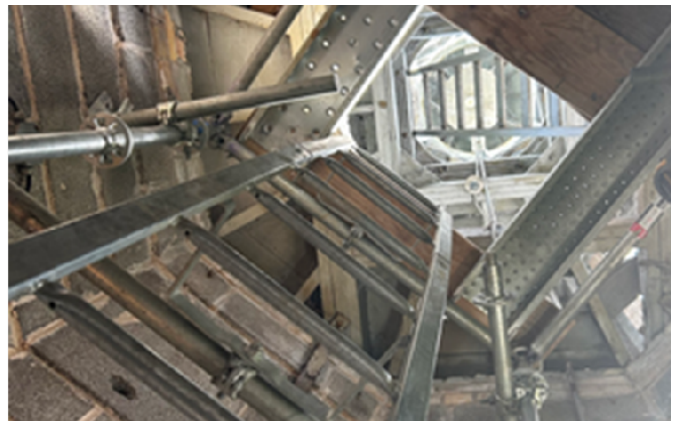
Scaffolding installation for access to top of lighthouse.
