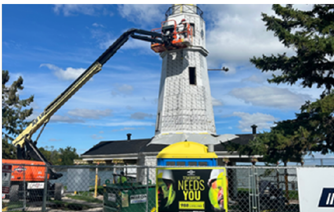
Exterior brick preparation.
