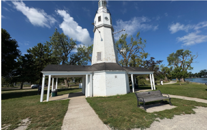
Kimberly Point Lighthouse prior to start of construction.
